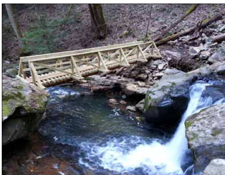
The new 28-foot-long bridge spanning McAlloyd Branch on the Fiery Gizzard Trail. Photo by Jason Reynolds.
