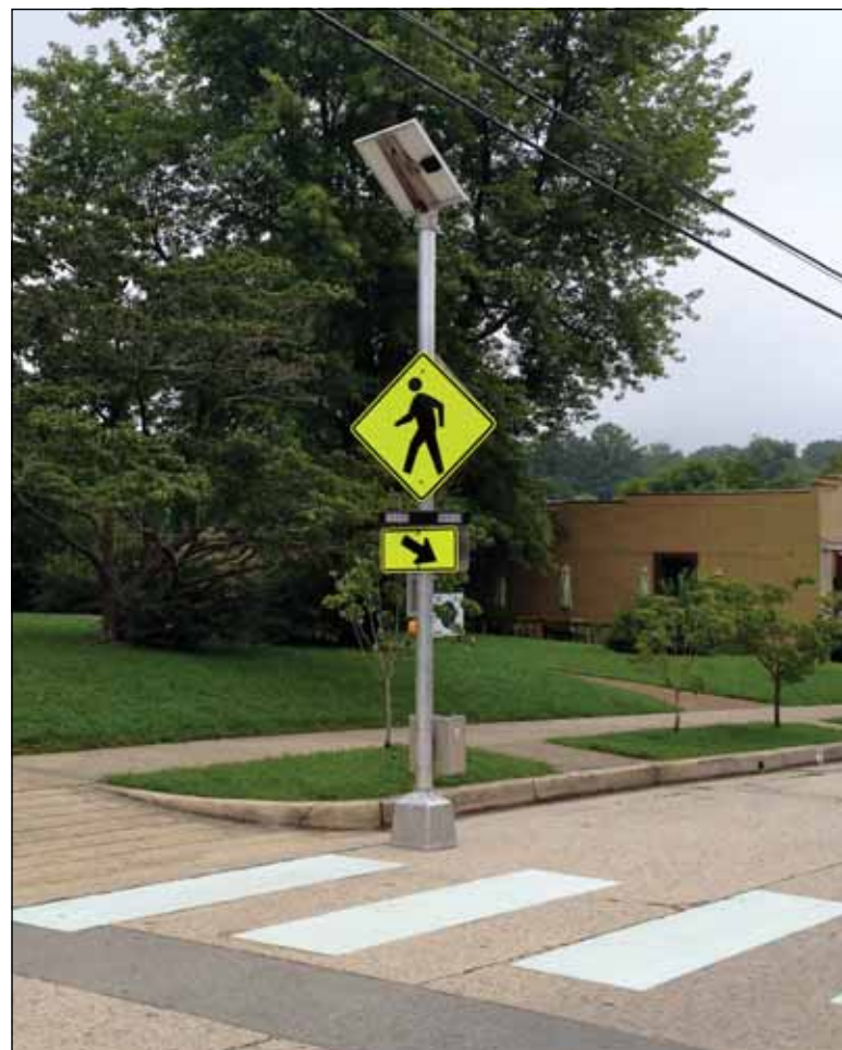
This is one of two solar-powered crosswalk warning lights on University Avenue that were installed by the Franklin County Highway Department in mid-July at the same time a crosswalk was painted on the street.
