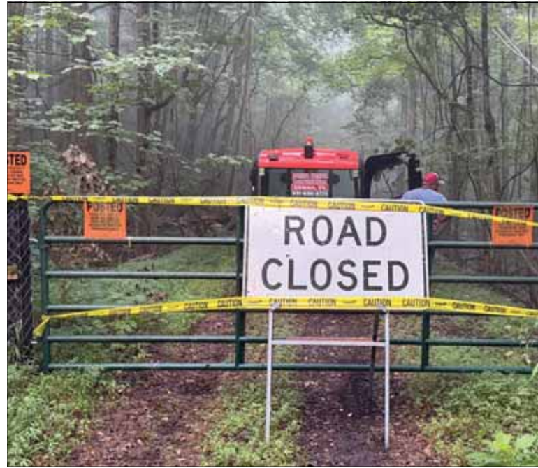
Dangerous construction phase. We know everybody's excited about the Mountain Goat Trail Sewanee-Cowan section, but for the rest of August (at least) we need everyone to steer clear of the railbed. We'll let you know soon when it's safe to be back on the section. Thanks for your cooperation!
